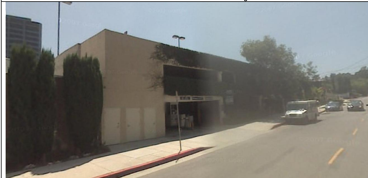
Subject Site's Parking Structure to South of Building
