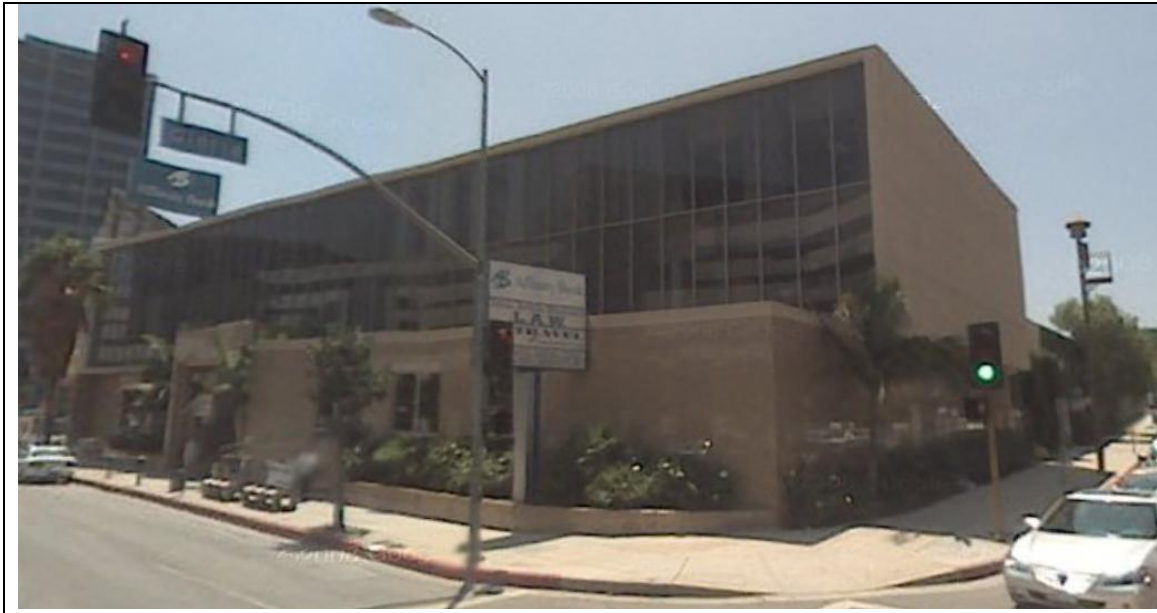
South East View of Subject Site
